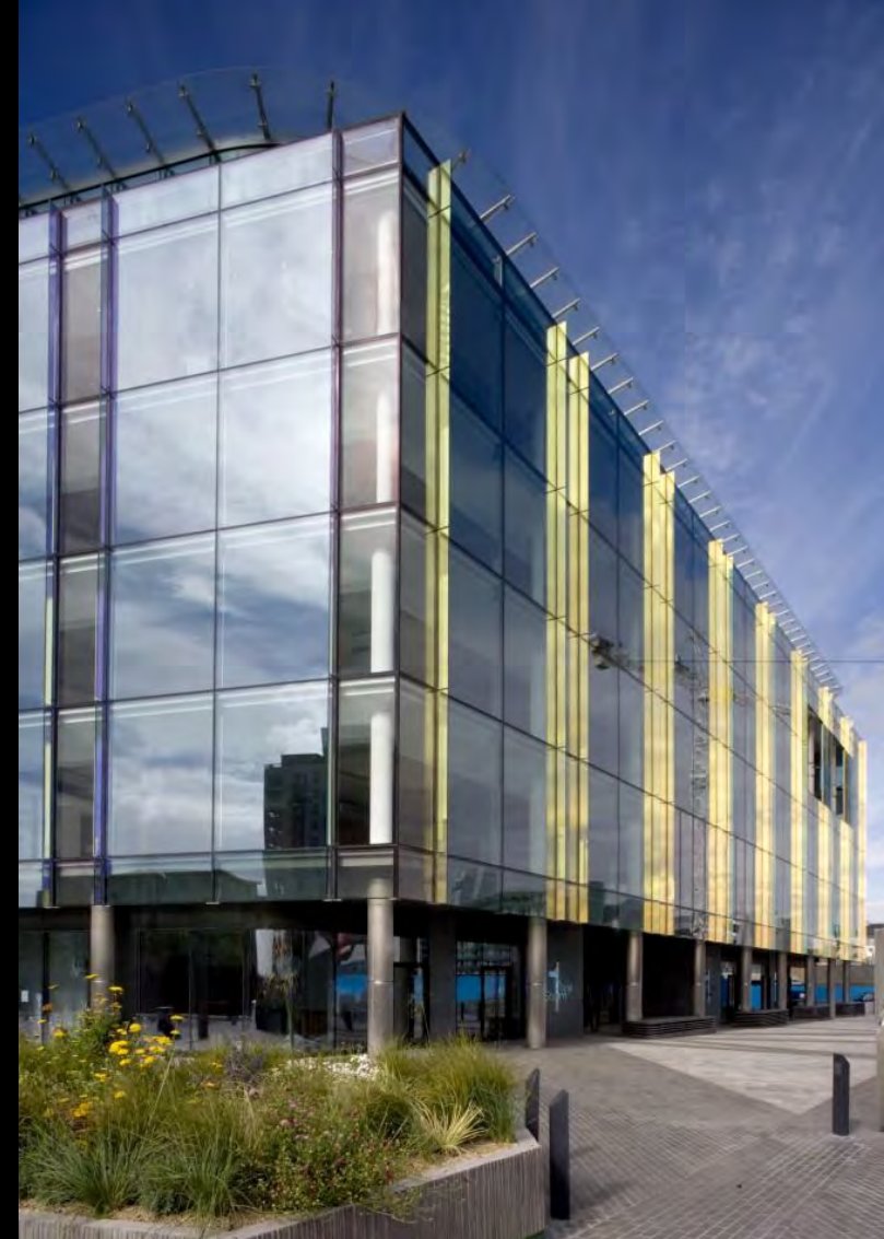
Grand Canal House, DMOD, 2007
