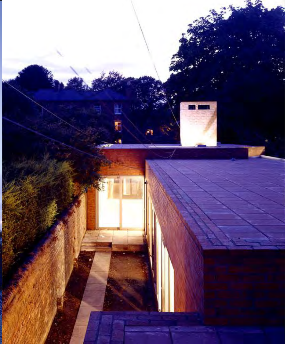
Brick House FKL 2001
