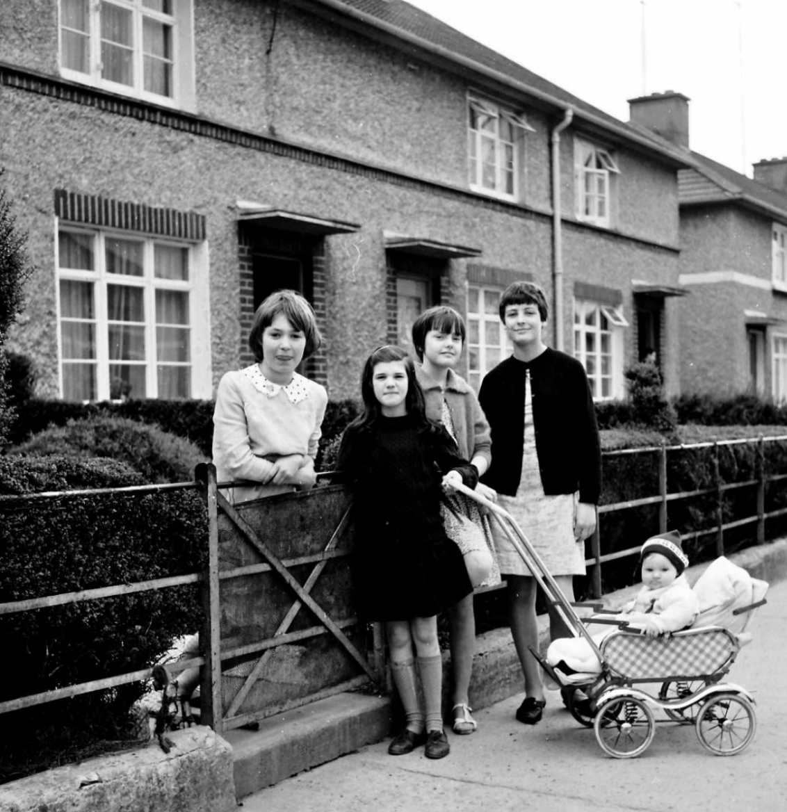
Ballyfermot Crescent HG Simms, Dublin Corporation Housing Architect 1947
